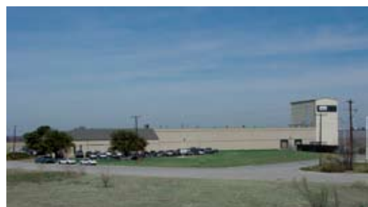
TexLoc Facility Fort Worth, Texas
